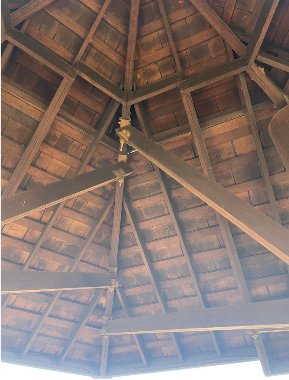
Underside of the Roof
