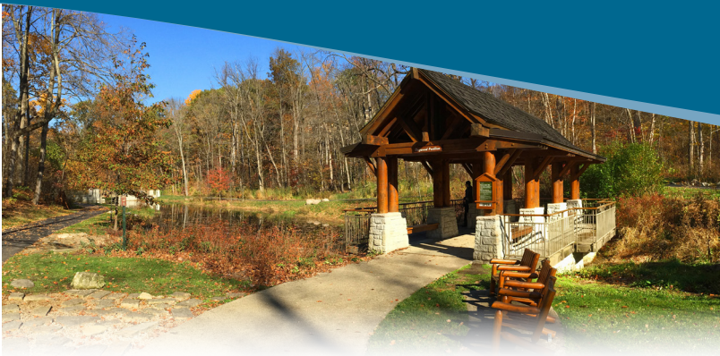
Adirondack-style shelter at Hills & Dales MetroPark
